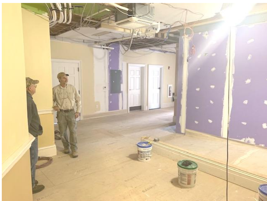
The hallway near the choir room and nursery is well underway! The elevator walls have been put up.
